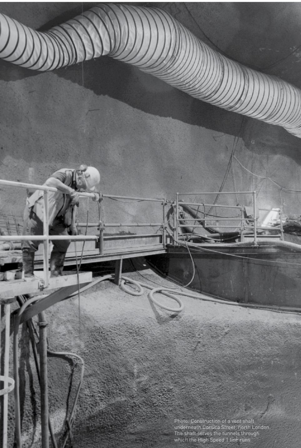
Photo: Construction of a vent shaft underneath Corsica Street, north London. The shaft serves the tunnels through which the High Speed 1 line runs.
