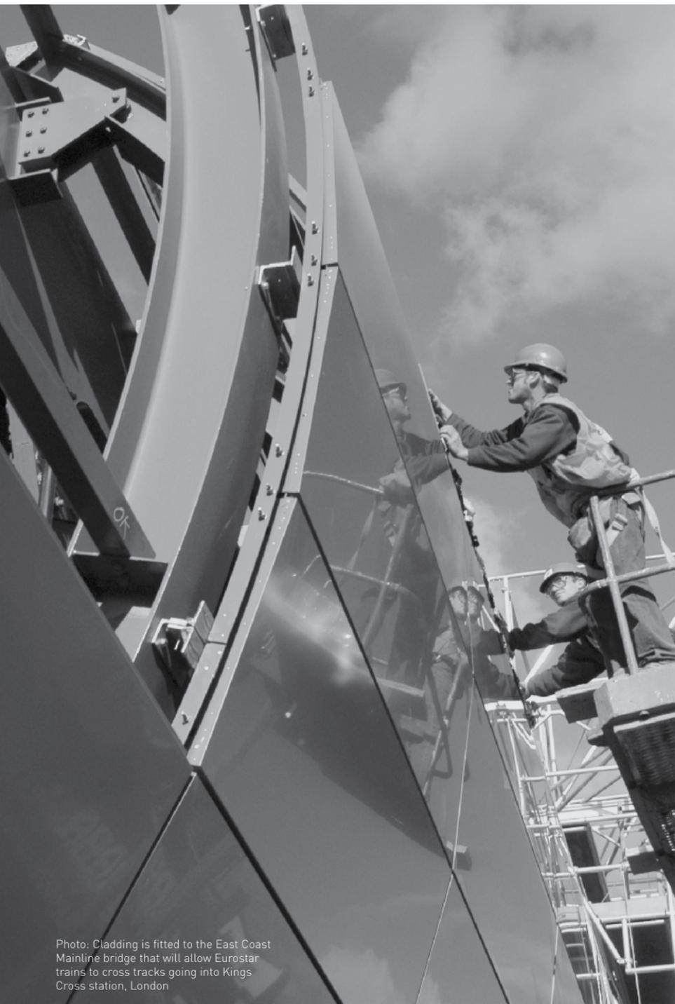
Photo: Cladding is fitted to the East Coast Mainline bridge that will allow Eurostar trains to cross tracks going into Kings Cross station, London
