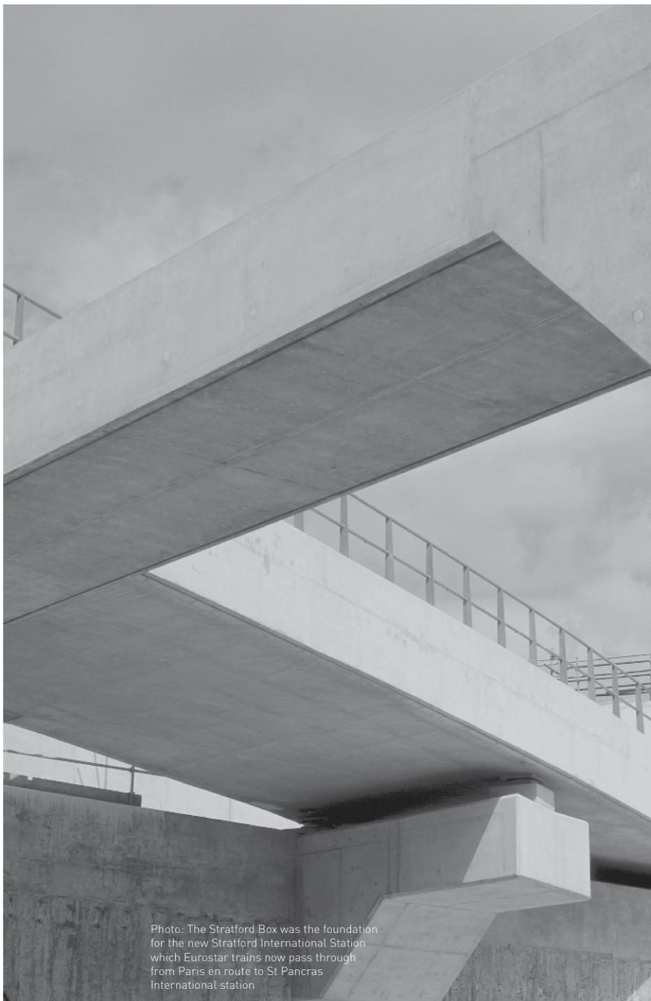
Photo: The Stratford Box was the foundation for the new Stratford International Station which Eurostar trains now pass through from Paris en route to St Pancras International station
